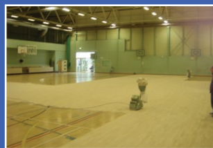
Sanding floor main sports hall
