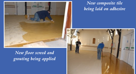
First coat of new floor seal being applied
